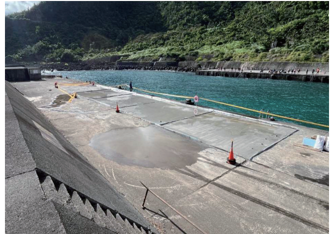
▲Figure 2-39 Restoration of the pier's concrete deck completed in July 2024
