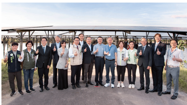
▲ Figure 2-15 Ta Ya Group's Zhiguang combined fish farm and solar power facility in Qigu District, Tainan City
