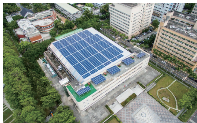
▲ Figure 3-3 National Sustainable Development Awards – Education Category Winner: National Chung Hsing University. The university has installed solar PV energy storage systems and EV charging stations on campus rooftops, advancing its goals of energy autonomy and net-zero carbon emissions
